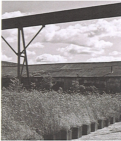
The Steel Yard, Providence, Rhode Island, 2010. The Steel Yard is a reclaimed urban landscape that represents the neighborhood's industrial history while also offering a campus for industrial-arts education, workforce training, and small-scale manufacturing.
